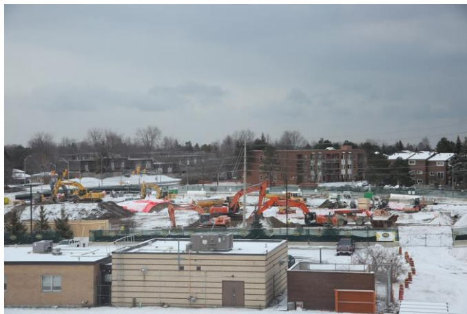
Construction of the long-term care home – February 2021
