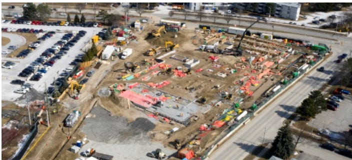
A look at the home's partially completed foundation on March 3
