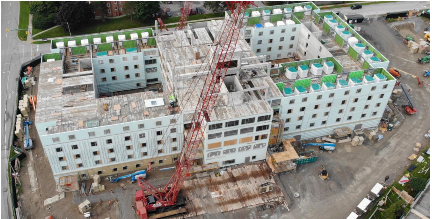
Crews working on the sixth floor on July 17, 2021
