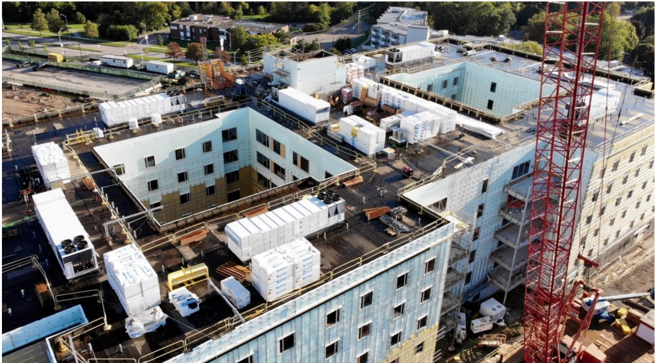
A look at the home's roof on September 26, 2021
