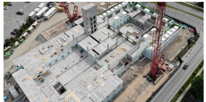
The partially completed third floor on May 21, 2021
