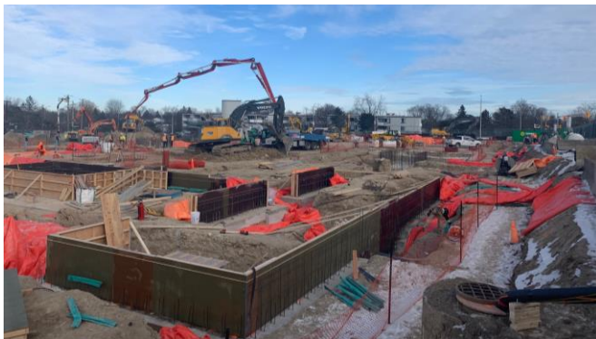
Foundational work on February 9, 2021
