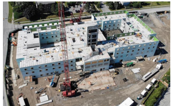
Crews working on the fourth floor on June 19, 2021
