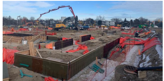
Foundational work on February 9, 2021
