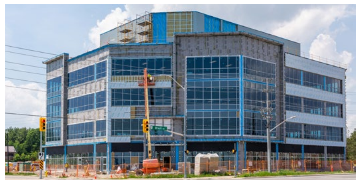
Construction progress on the Jerry Coughlan Health & Wellness Centre in May 2022.
