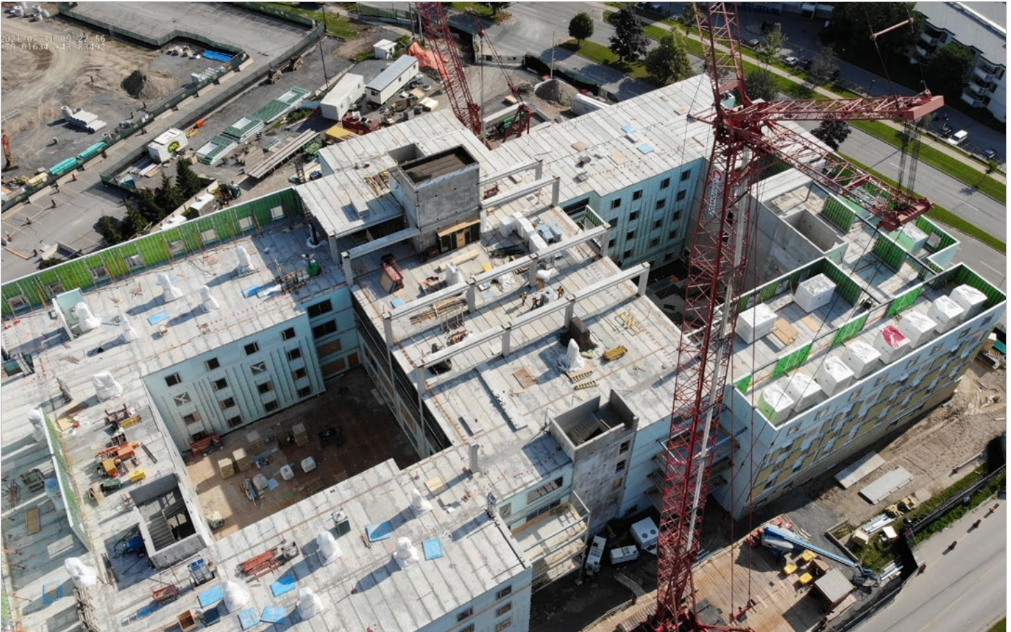
Construction of Lakeridge Gardens in July 2021.
