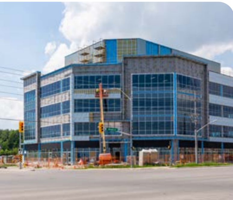
Construction of the Jerry Coughlan Health & Wellness Centre.
